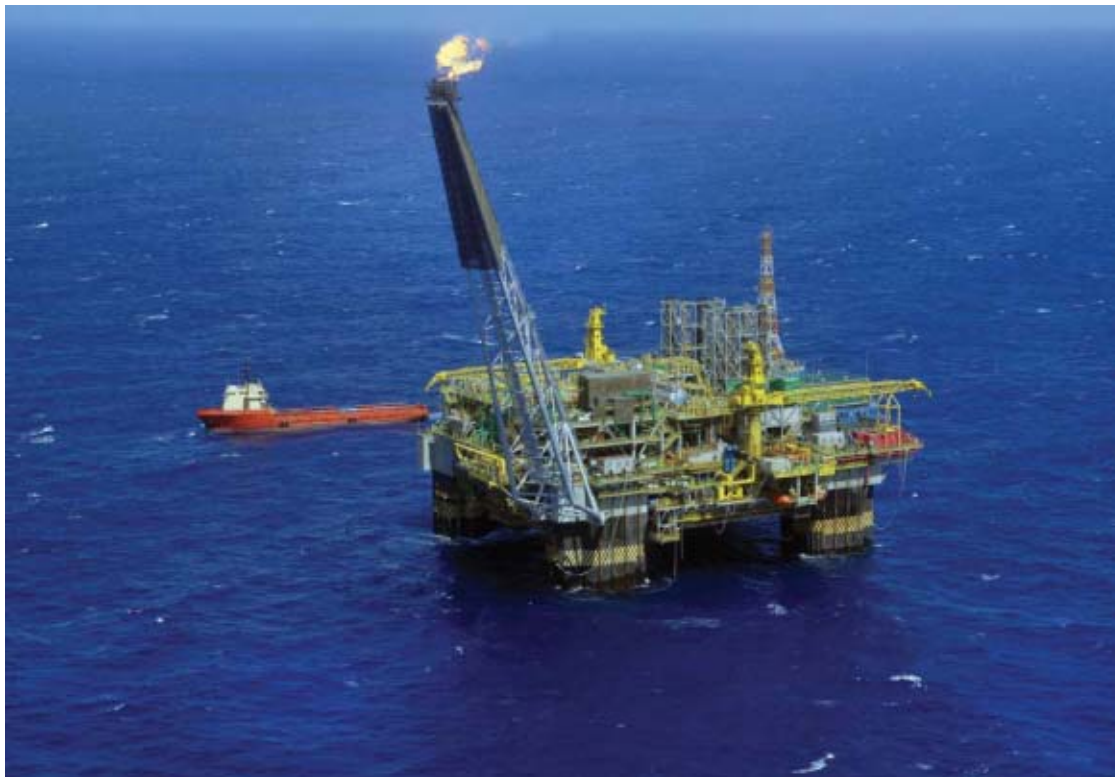
The P-52 semisubmersible production unit in the Roncador field off Brazil has designed processing capacity of 180,000 bo/d (Fig. 4). Photo from Petrobras.
