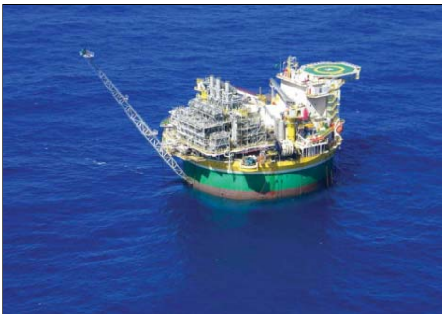
Petrobras installed the world's first cylinder-shaped FPSO in the Pirama field off Brazil (Fig. 3). Photo from Sevan Marine ASA.
